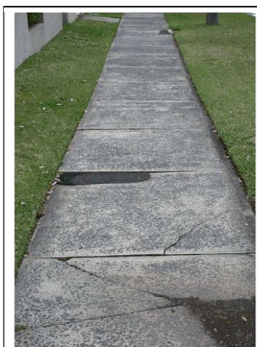
Footpath in fair condition (5 to 6 rating).
