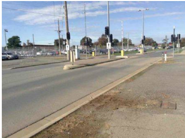
Existing crossing boom gates
