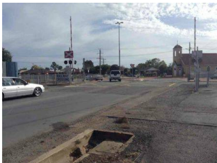
View toward west and railway crossing
