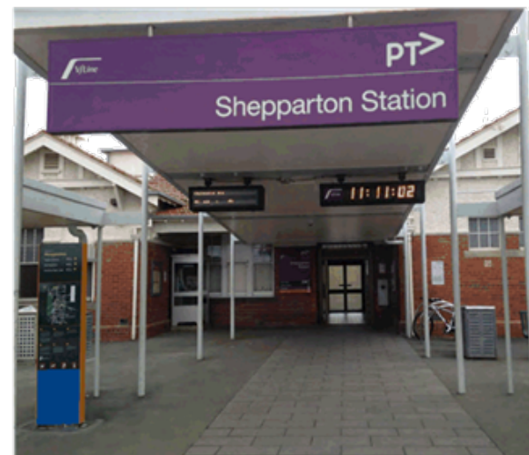
Shepparton Railway Station Entrance
