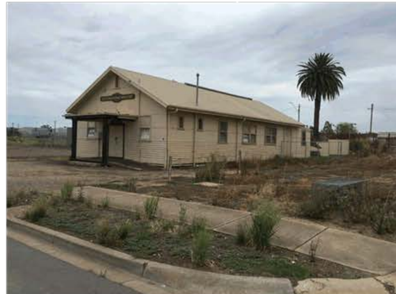
Figure 14 Building No.19 The Victorian Railway Institute Hall
