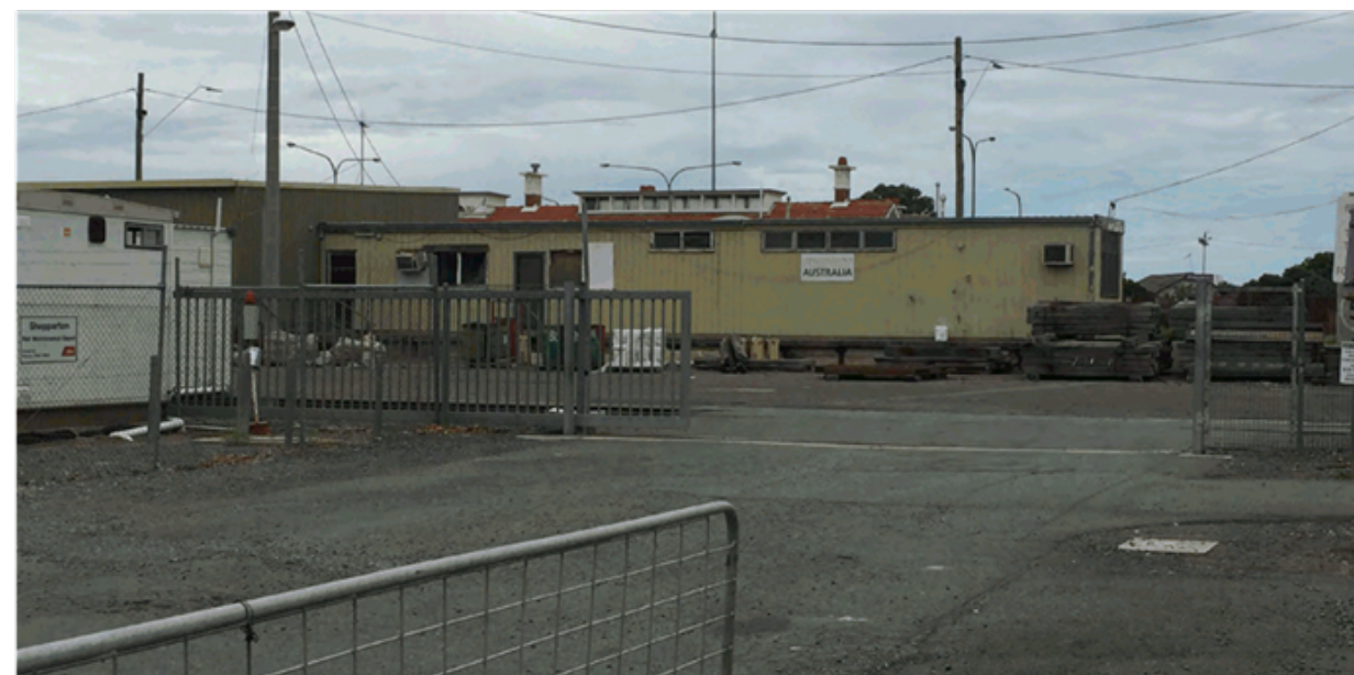
Figure 9 Building No.9 Demountable ex-LCL portacabin building off Hoskin Street (near Vaughan Street)
