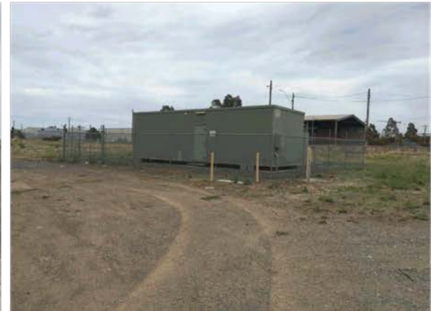
Figure 15 Building No.20 High security fenced and windowless electrical substation off Purcell Street (for supplying V/Line signaling power)
