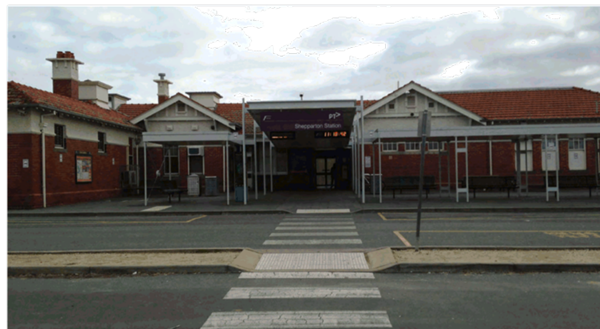
Shepparton Railway Station Entrance
