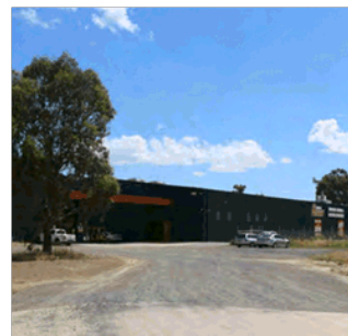
Unfinished or poorly maintained driveways with gravel spill into the public realm (inappropriate materials)
