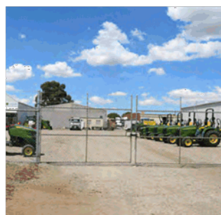
Avoid: Areas of car parking/ hardstand stock display that are not softened by a landscape buffer when viewed from the road
