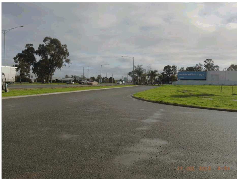
Numurkah Road service lane looking north
