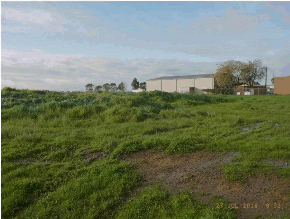
Stockpiling on the child care centre site
