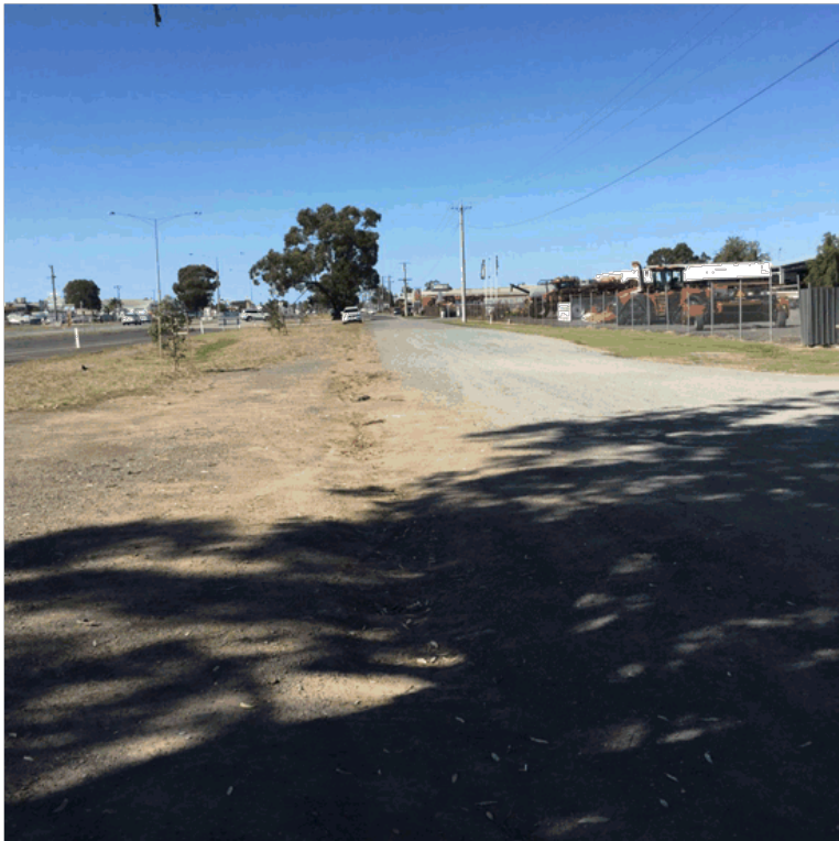
Existing gravel service road connecting the properly made service road to the Advance Fitness gym
