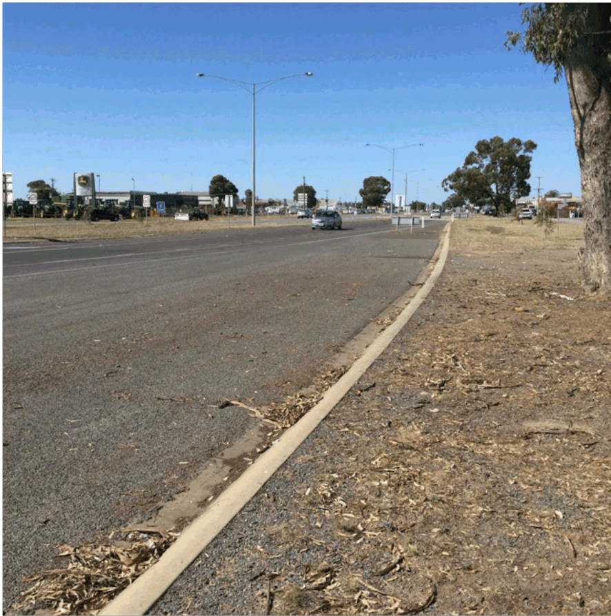
Existing unused pavement on Numurkah Road which could be utilised for a left turn lane into the gym
