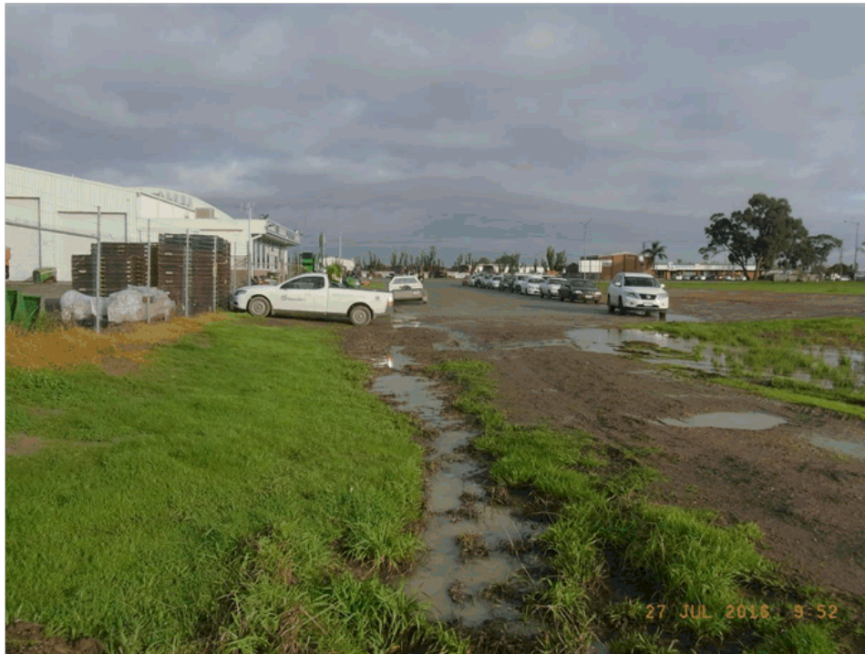
Open drain to the pit
