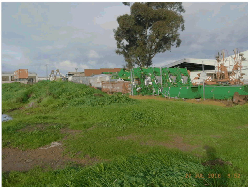
Stockpiling on the child care centre site
