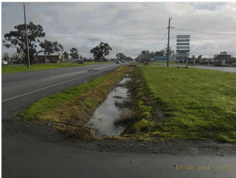
Open drain looking north
