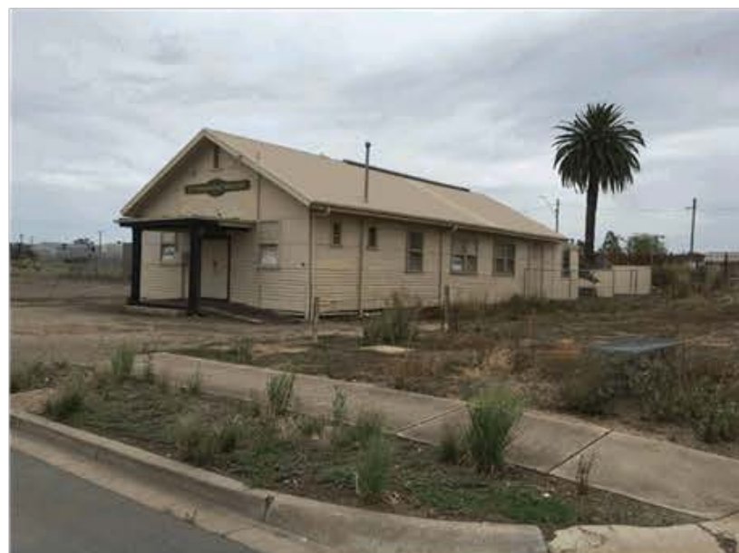
Figure 14 Building No.19 The Victorian Railway Institute Hall
