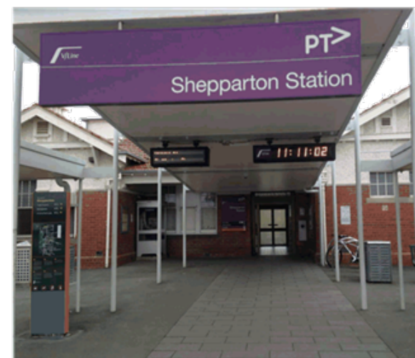
Shepparton Railway Station Entrance
