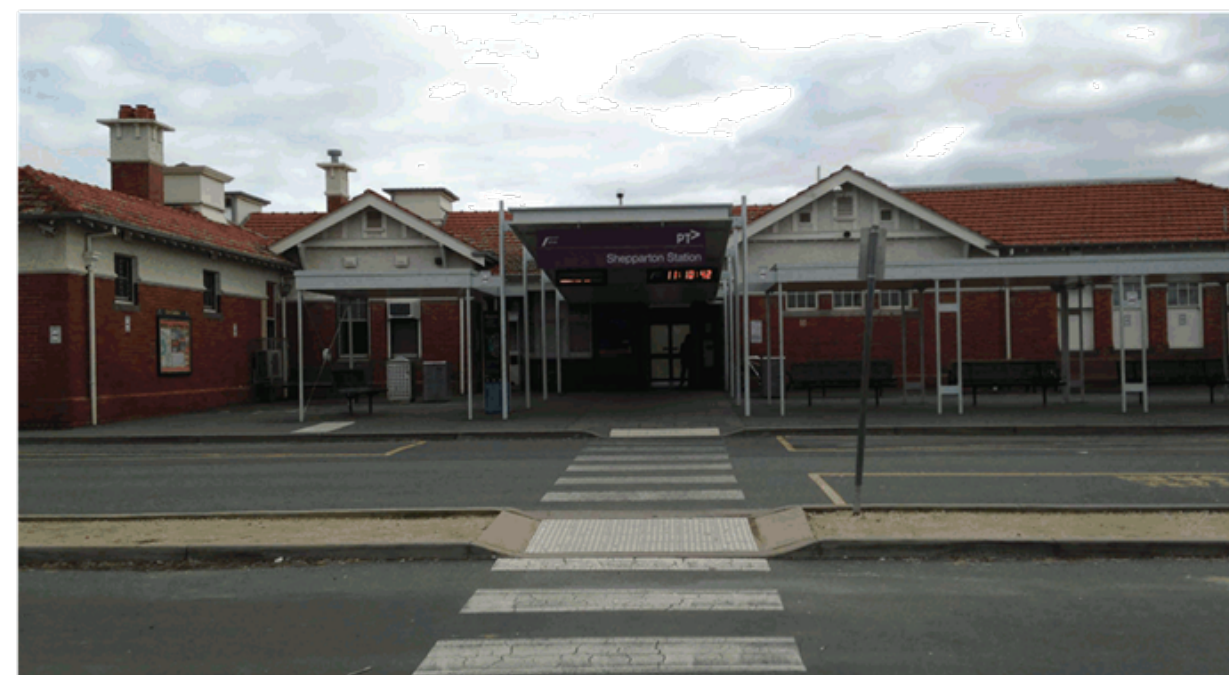
Shepparton Railway Station Entrance
