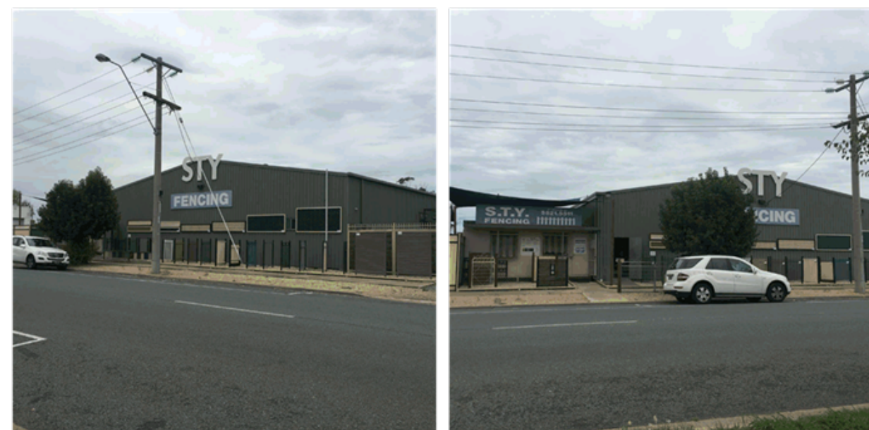
Figure 7 Building No.6 Sty Fencing warehouse and yard on Hoskin Street
