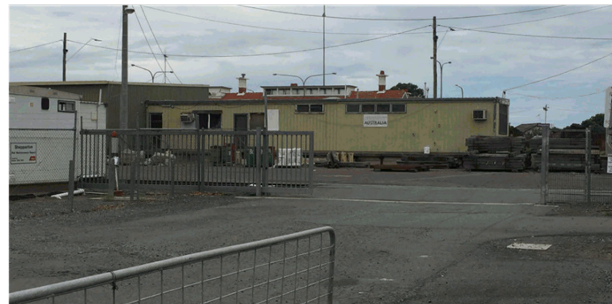
Figure 9 Building No.9 Demountable ex-LCL portacabin building off Hoskin Street (near Vaughan Street)
