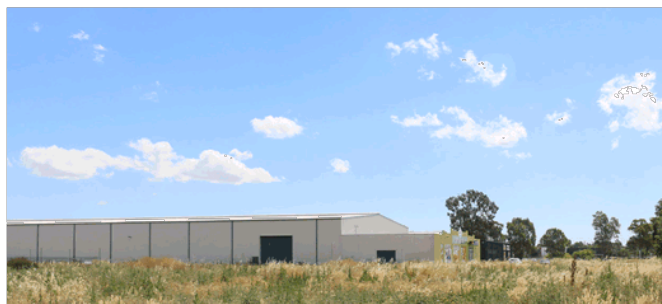
Avoid: Large, blank façades and use of bright, eye catching colours that are not sensitive to the residential area nearby
