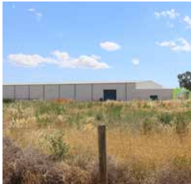
Development and hard stand car parking constructed to lot boundaries without provision for landscaping
