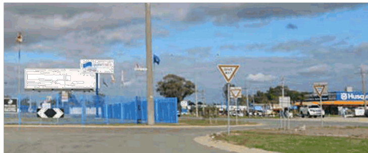
Disorganised advertising, road and directional signage: visual clutter with limited visual hierarchy for road users
