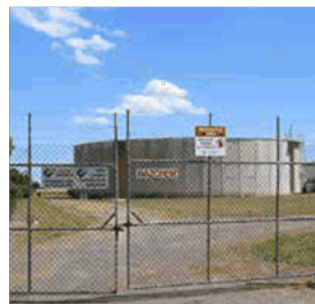
Scale and siting of existing industrial uses adjacent to residential area creates interface issues.
