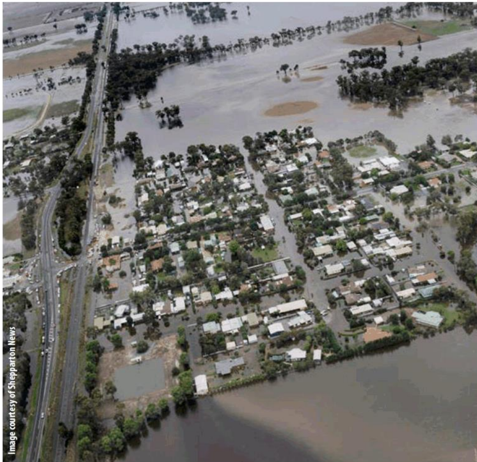
Aerial view of flooding at Tallygaroopna in March 2012 (source: Tallygaroopna Local Flood Guide, December 2016)
