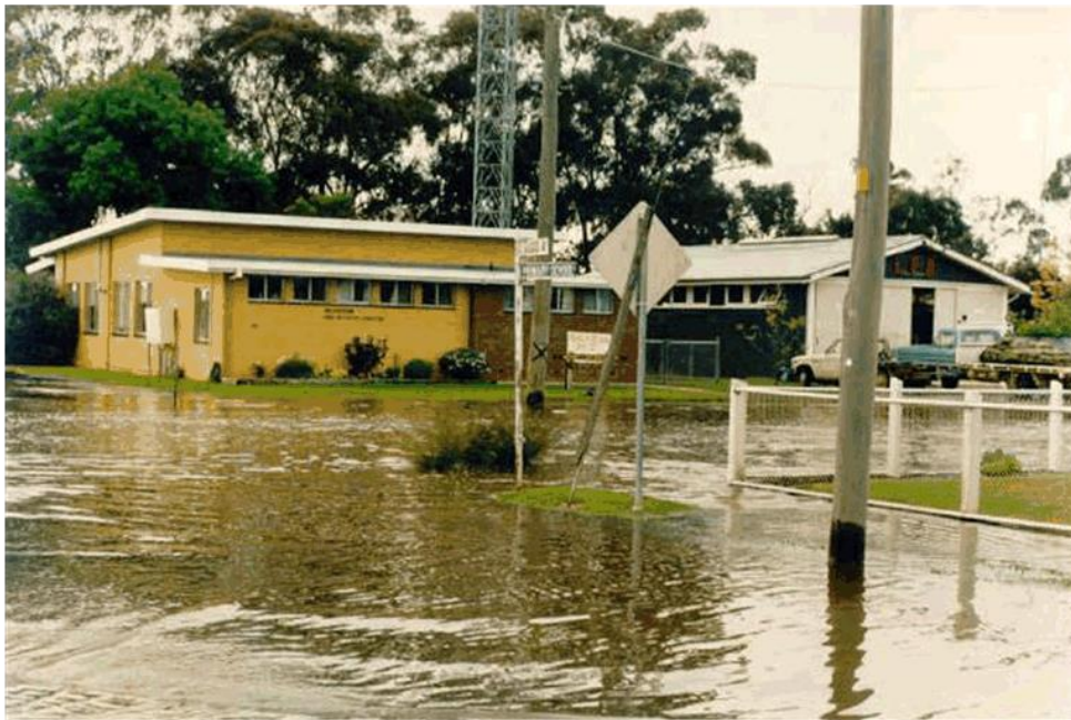
Flooding at corner of Judd and Waverley Avenues, October 1993 (source: WBM, 2005)
