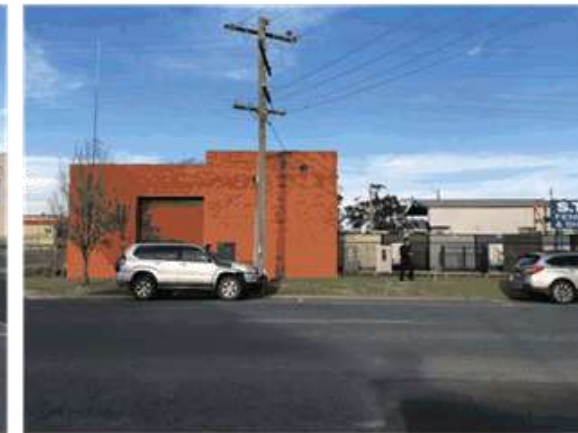
2. Close-up view from Vaughan St West - Existing brick building to be demolished for new entry to pedestrian overpass
