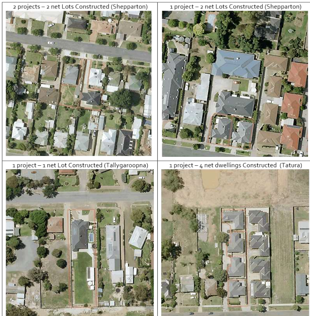
Image 2: Dispersed Infill Lot Construction – City of Greater Shepparton
