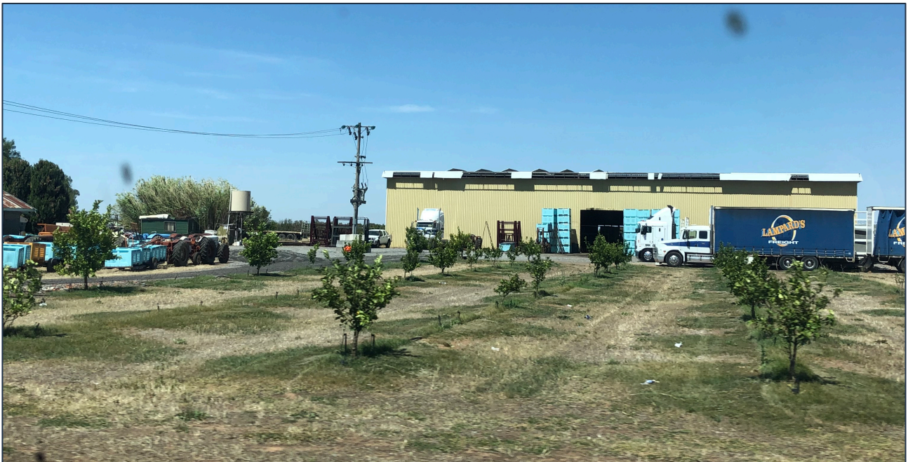
Coolstore and packing sheds (RMCG)
