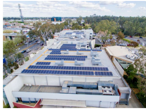
Figure 12: Solar panels installed at Council's Welsford Street offices in 2018
