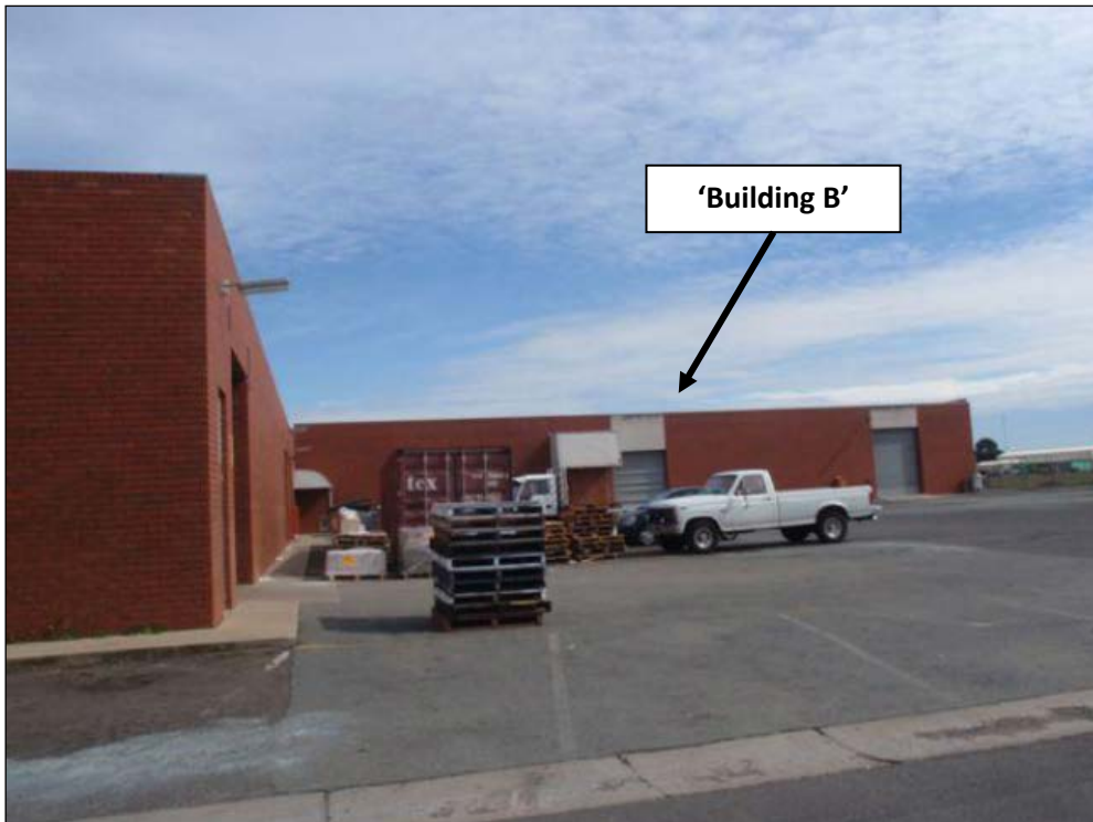
Figure6: View to Beaumont Tiles loading area and the common property.
