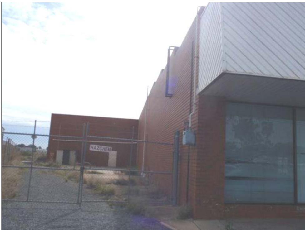
Figure 4: View along the western elevation of the existing buildings.
