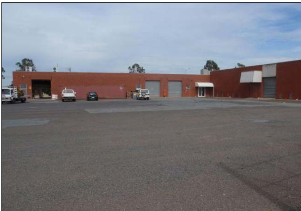
Figure 7: View to the northern and eastern elevations of the existing buildings.
