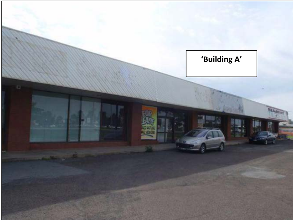
Figure 3: Benalla Road frontage of the existing building.
