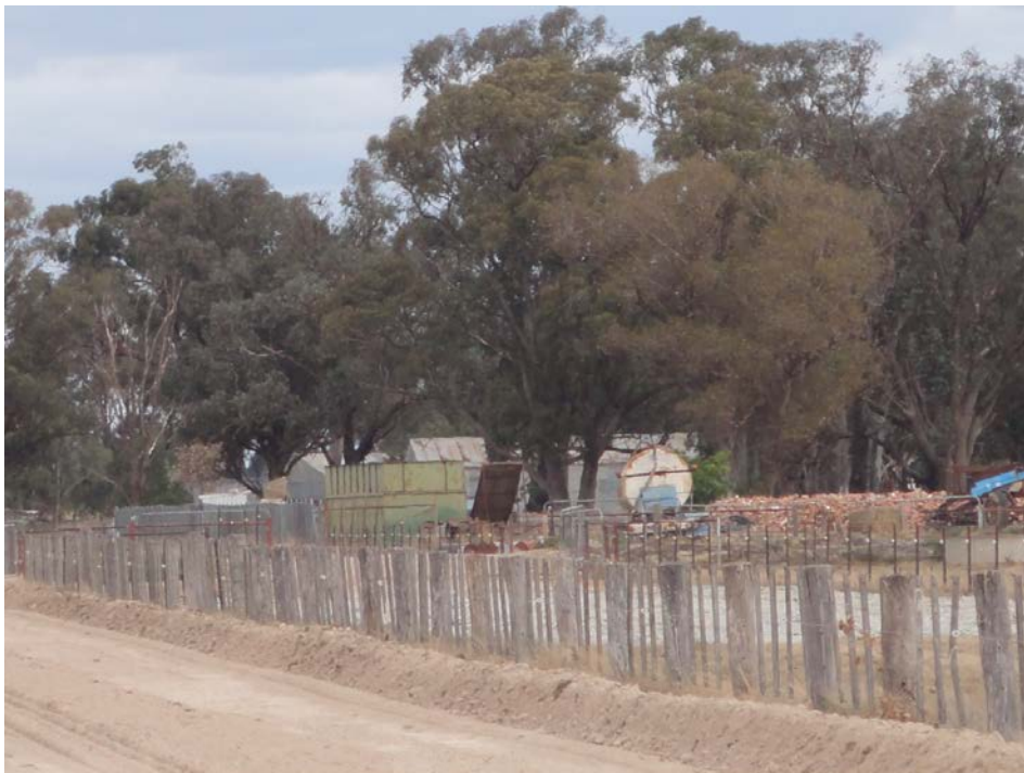
Equipment and stockpiles of bricks
