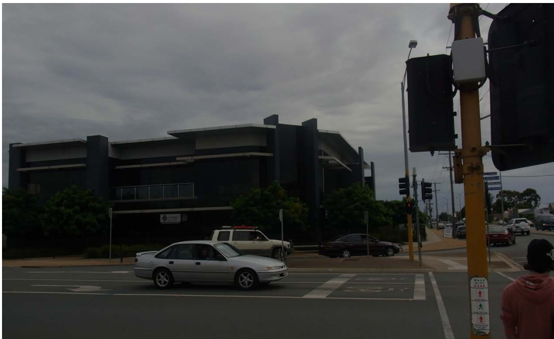
View of building looking north across Knight Street
