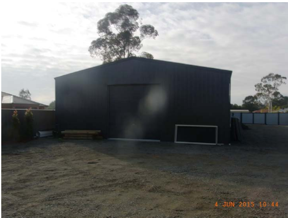
Photo 3 above: View of the rear of the shed
