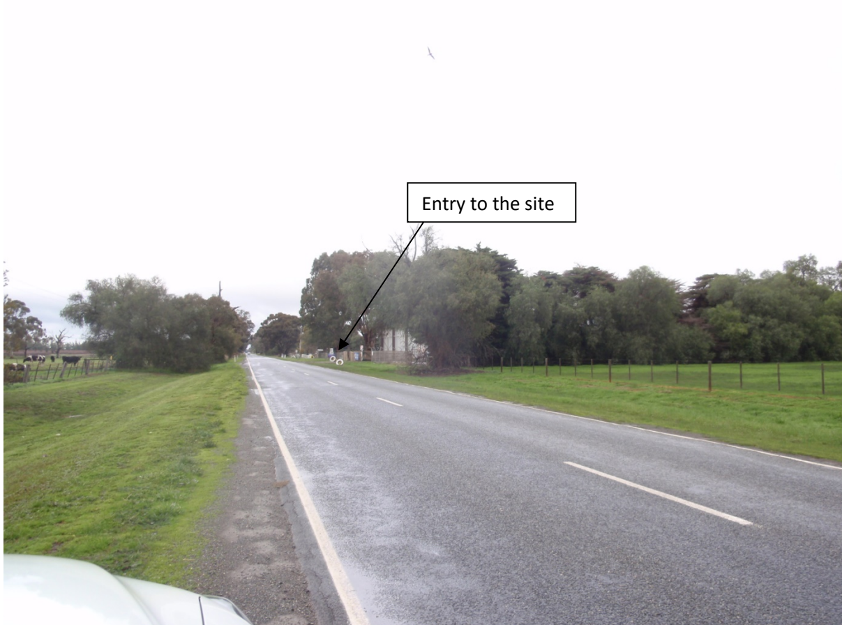
Looking south along Toolamba Road.
