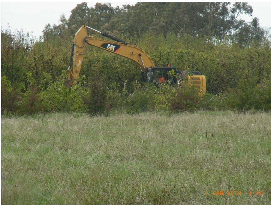
Excavator on eastern end of land removing orchard trees
