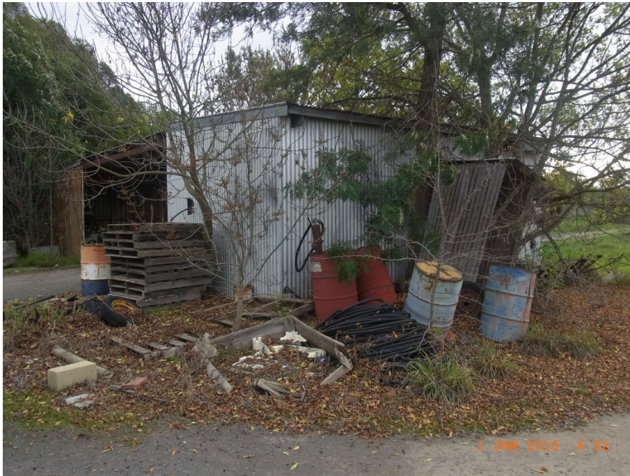
Looking west at packing shed, showing old fuel drums and pallets.
