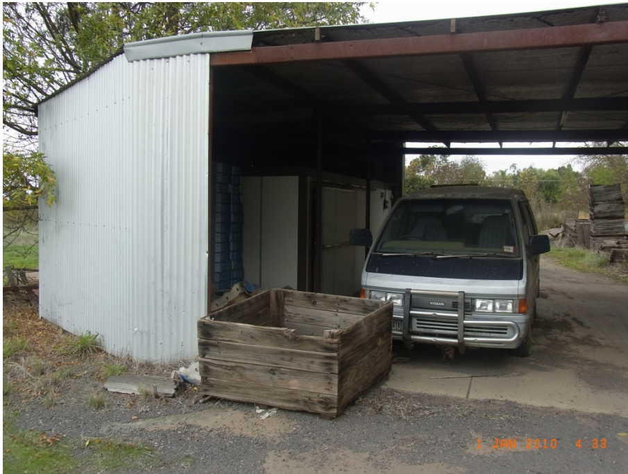
Looking south into packing shed showing cool store on left side
