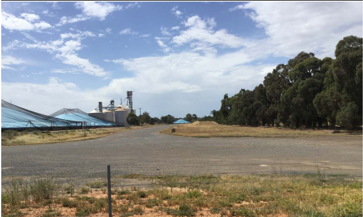
Above photo shows internal access way
