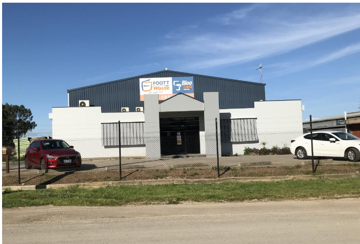
A photo of the existing Foott Waste Facility in Carroll Road.
