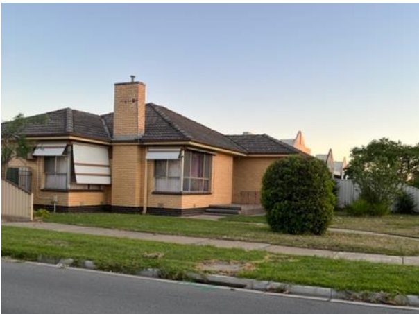
View of existing dwelling that is proposed to be demolished to make way for the petrol station
