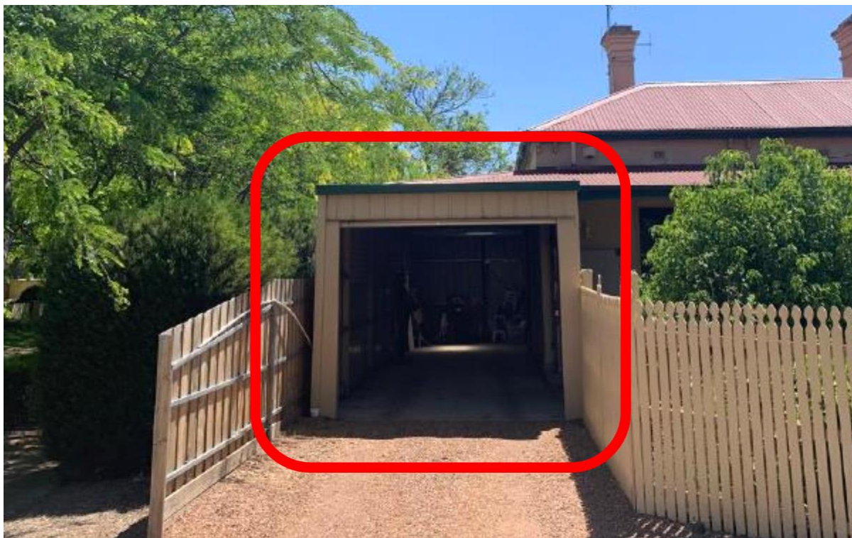
Existing garage to be demolished
