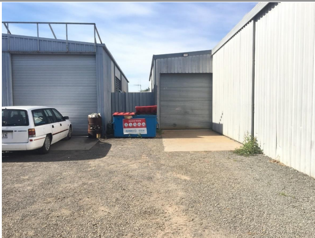
Proposed boundary fence to be constructed where the skip bin is located
