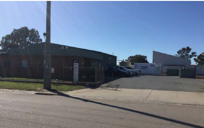
Office space for Downer
