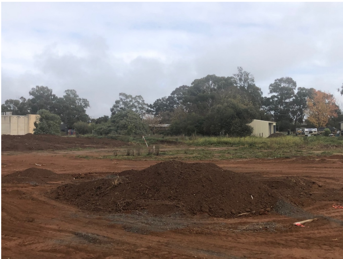
Rear view of subject land – photo taken from new subdivision (Apricot Court)
