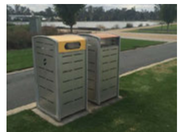
Bins on concrete slab example
