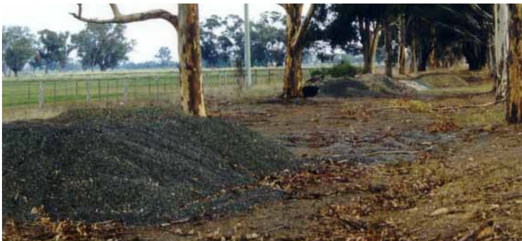
Figure 21 Roadside Construction Materials dumped under planted Avenue trees
