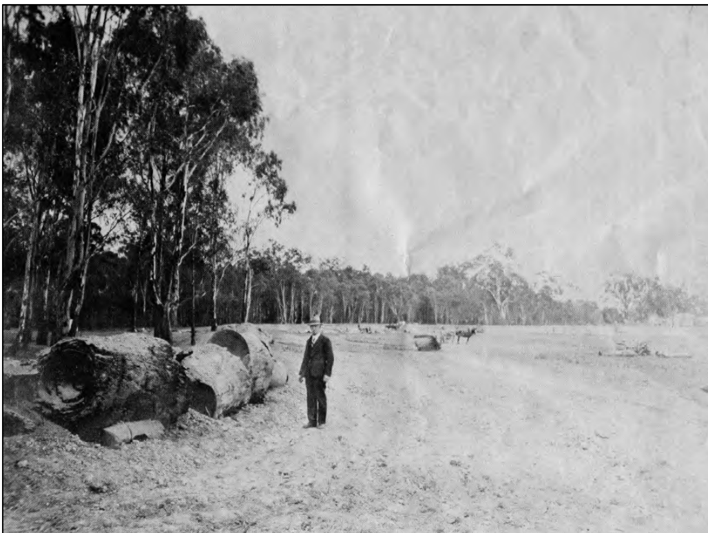
Clearing the lake bed, Victoria Park 1929, (Cr. John Pick)
